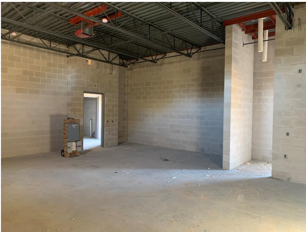
16. Locker Room Building – Interior CMU walls installed.
