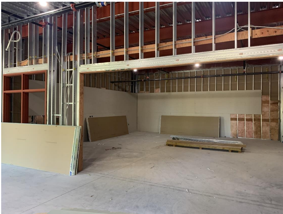
46. Area 4 West – Gyp board and sprinkler piping install in first floor classrooms in progress.
