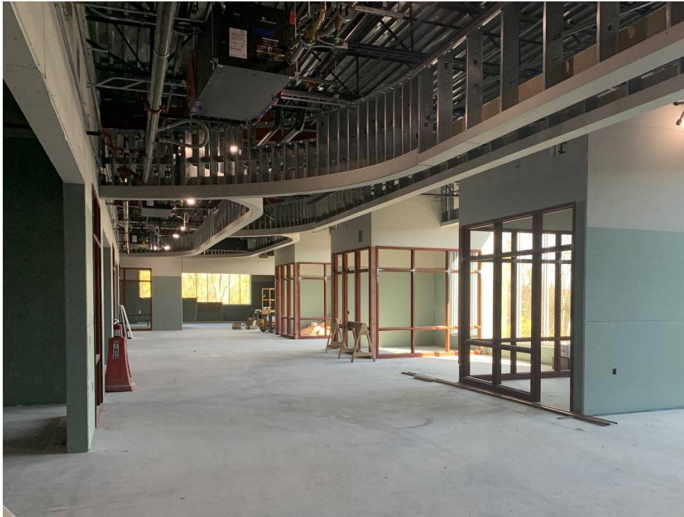
40. Area 4 East – Ceiling soffits in collab area in progress.
