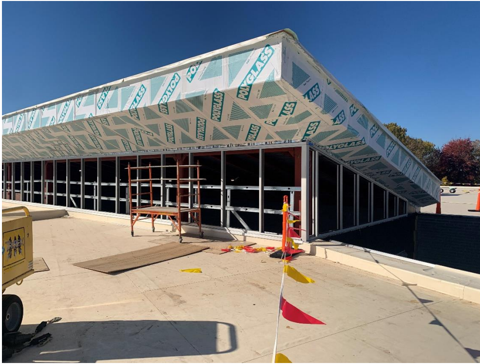
18. Area 1A Clerestory – Weatherproofing membrane installed. Curtain wall framing install in progress.
