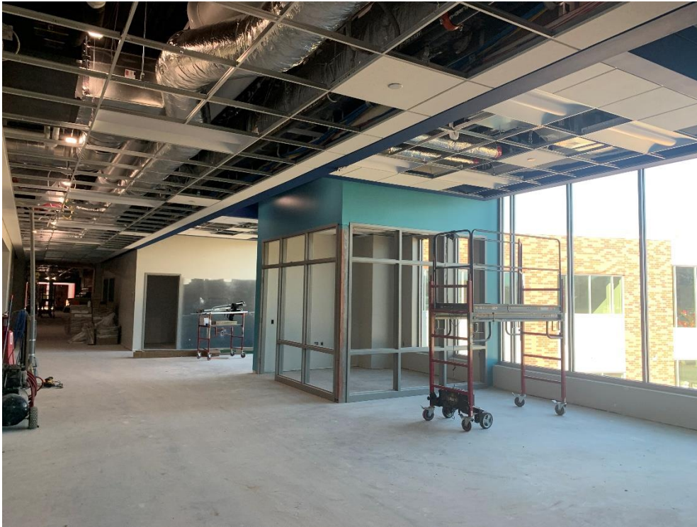
24. Area 6 North – Second floor classroom ceiling grid and electrical fixtures install in progress.
