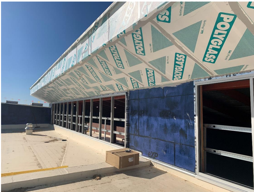
18. Area 1A Clerestory – Weatherproofing membrane installed. Curtain wall framing install in progress.
