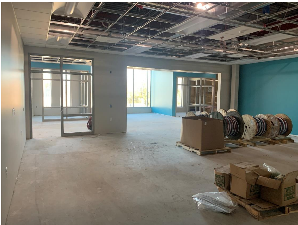
24. Area 6 North – Second floor classroom ceiling grid and electrical fixtures install in progress.
