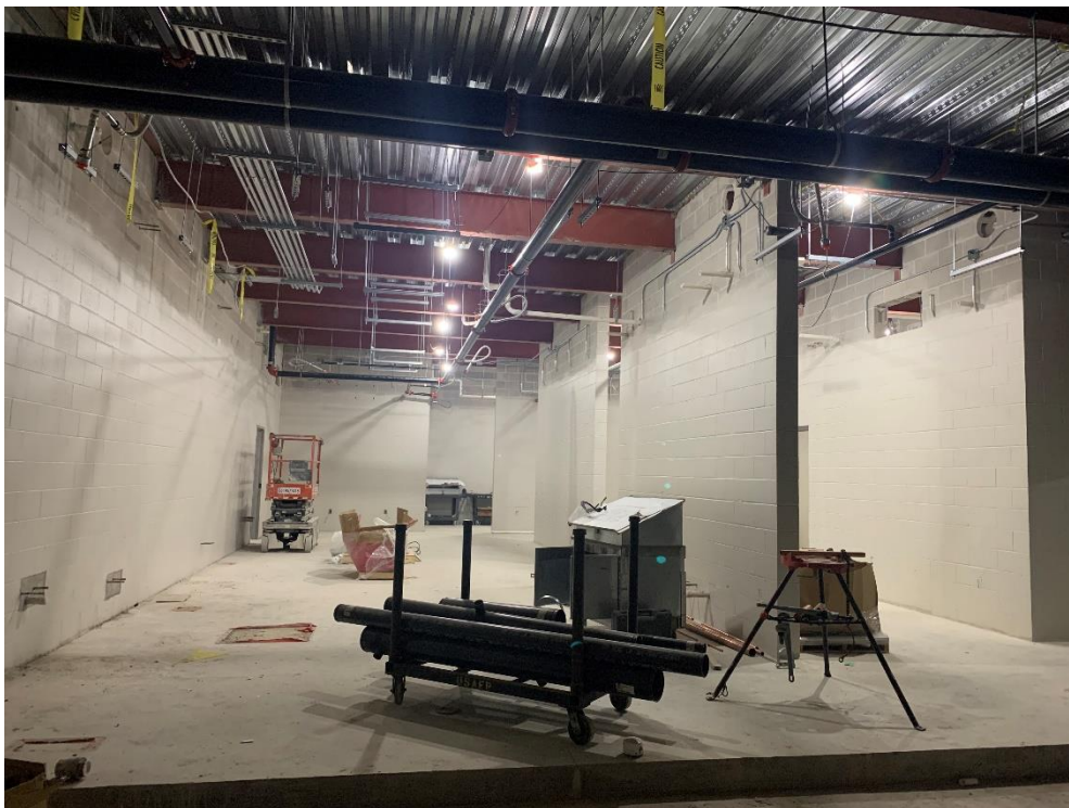
48. Area 3 – Kitchen sprinkler piping and above ceiling MEP install in progress.
