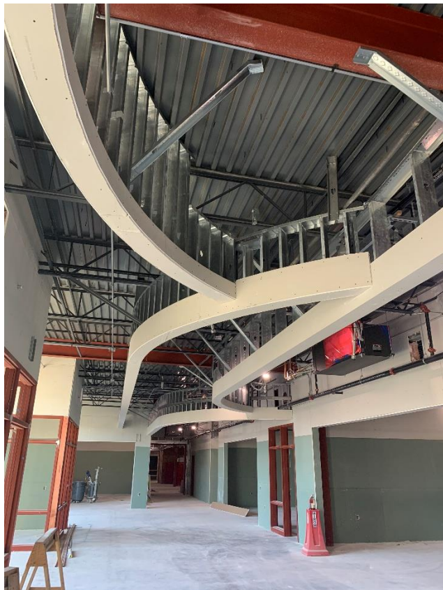
40. Area 4 East – Ceiling soffits in collab area in progress.
