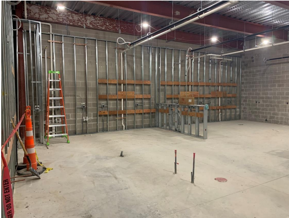
48. Area 3 – Kitchen sprinkler piping and above ceiling MEP install in progress.
