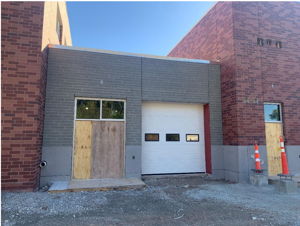
10. Area 3 West – Receiving overhead door installed. Storefront framing, glazing, and door install in progress.
