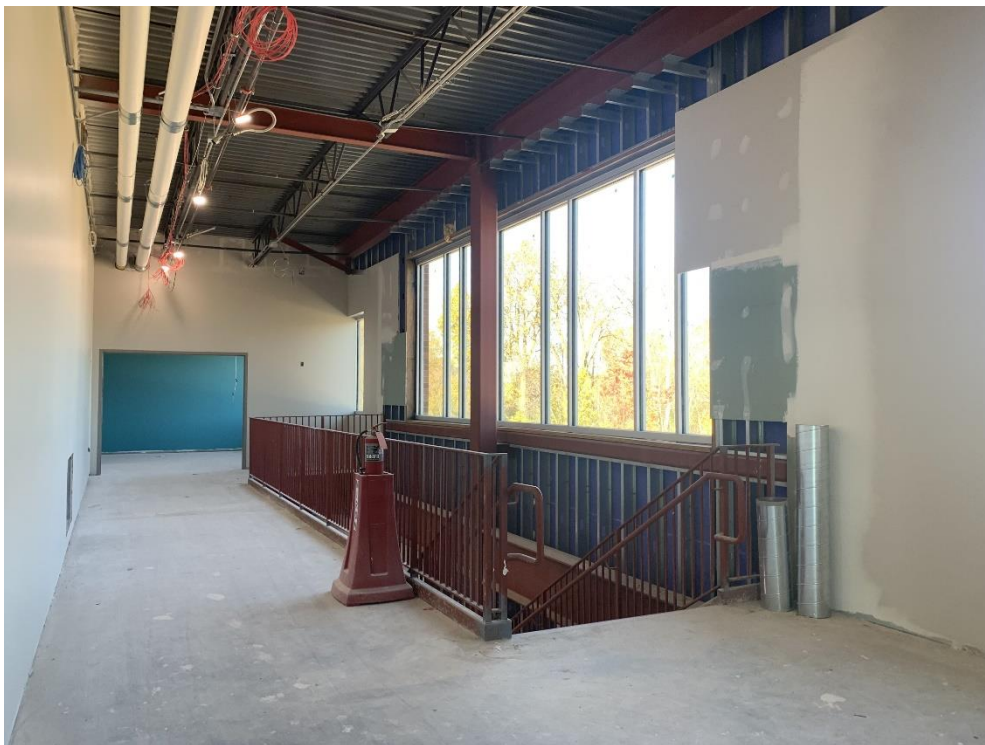
28. Area 5 – Second floor stair well gyp board, above ceiling MEP, and painting in progress.
