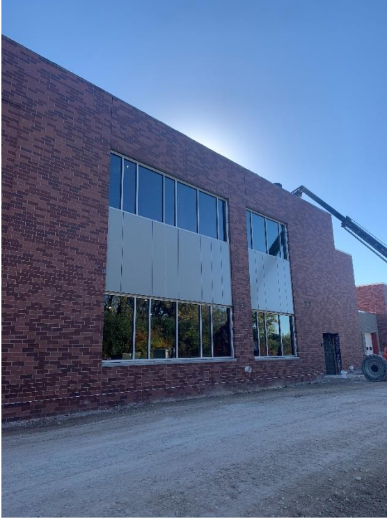
10. Area 3 West – Receiving overhead door installed. Storefront framing, glazing, and door install in progress.
