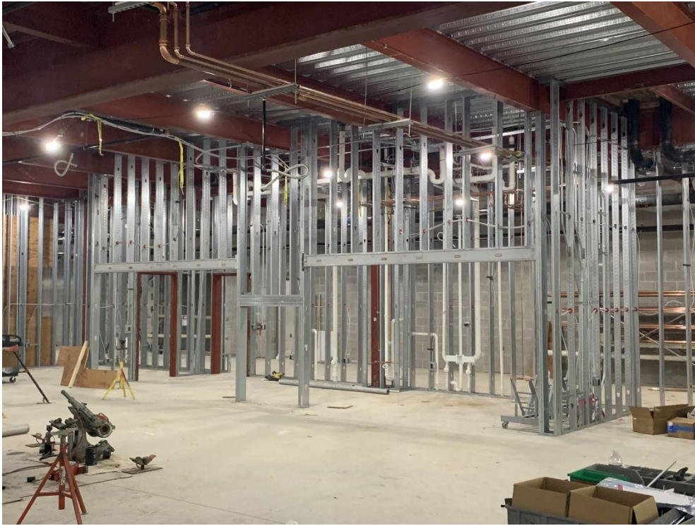
44. Area 3 – Wood blocking, gyp board, and sprinkler piping install in first floor flex cafe in progress.
