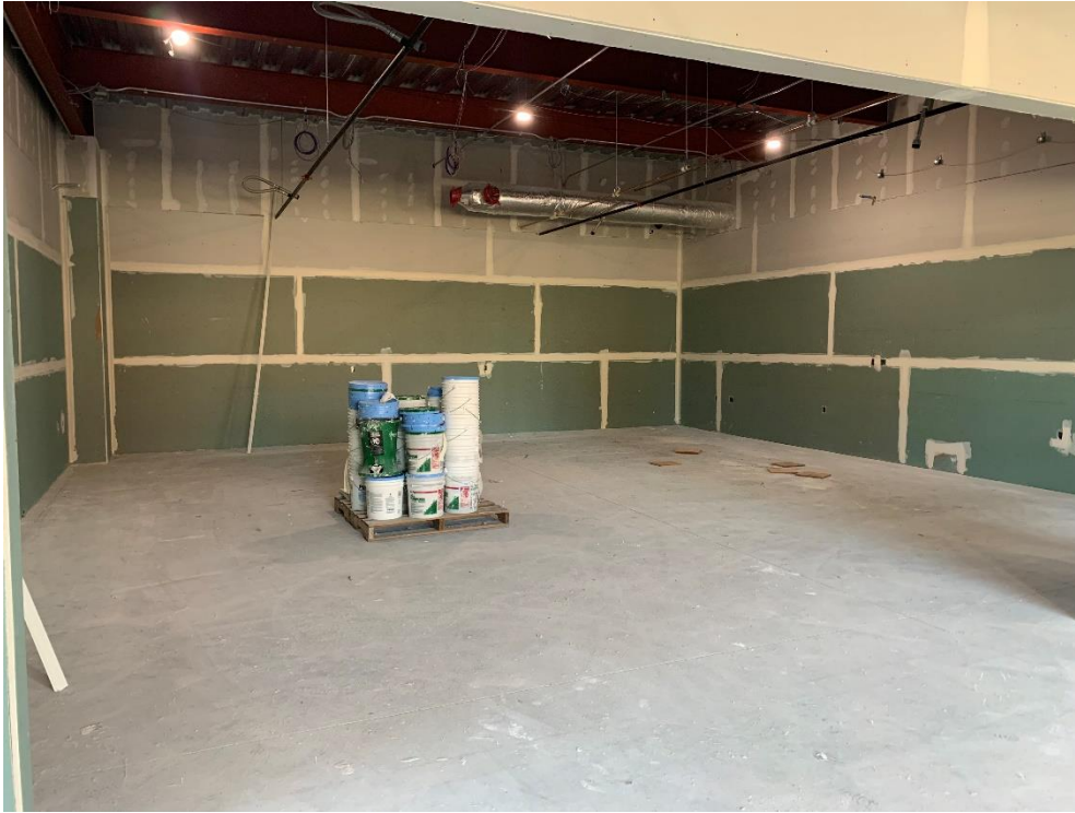
36. Area 5 – Gyp board, taping, mudding, and above ceiling MEP install first floor flex café in progress.
