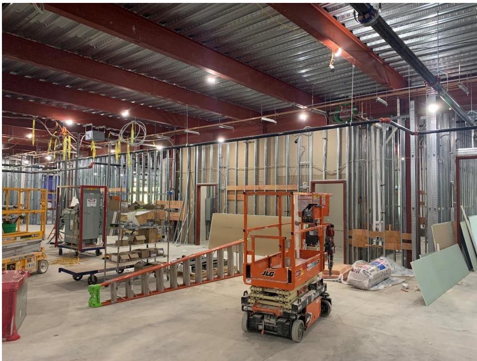
44. Area 3 – Wood blocking, gyp board, and sprinkler piping install in first floor flex cafe in progress.
