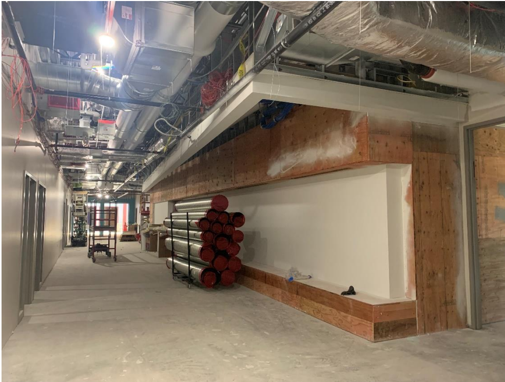
26. Area 5 East – Collab area above ceiling MEP install in progress.
