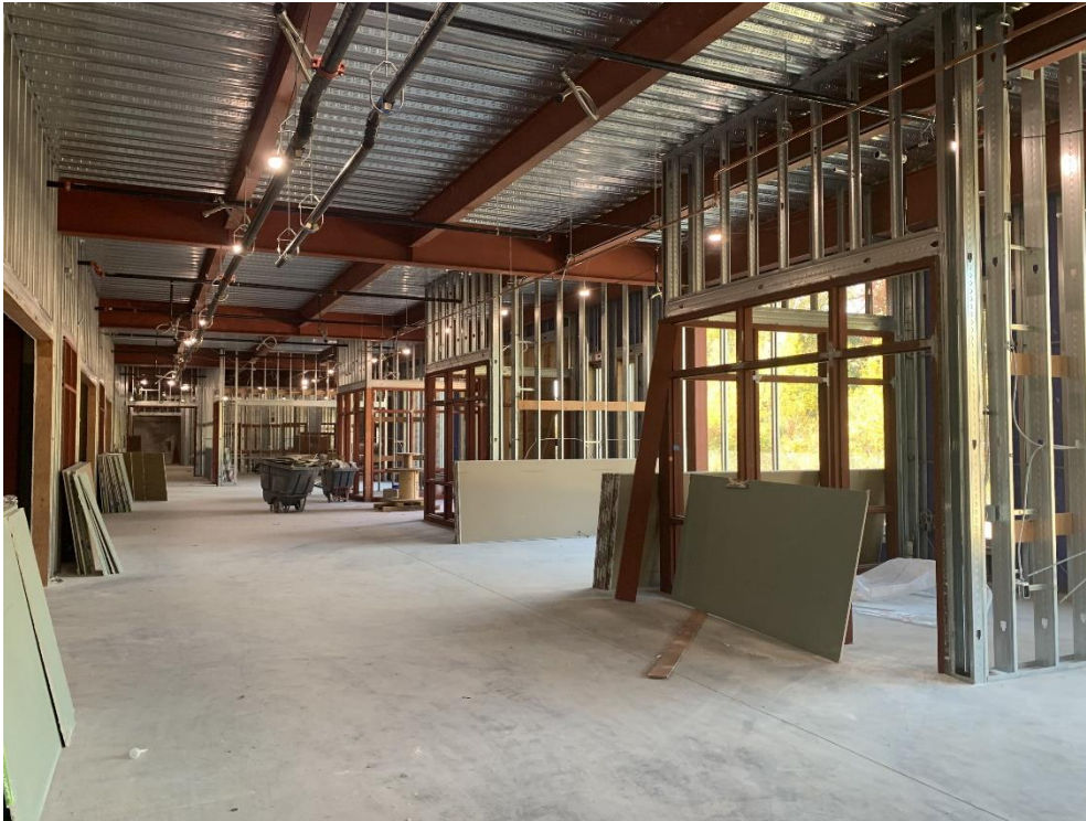
46. Area 4 West – Gyp board and sprinkler piping install in first floor classrooms in progress.
