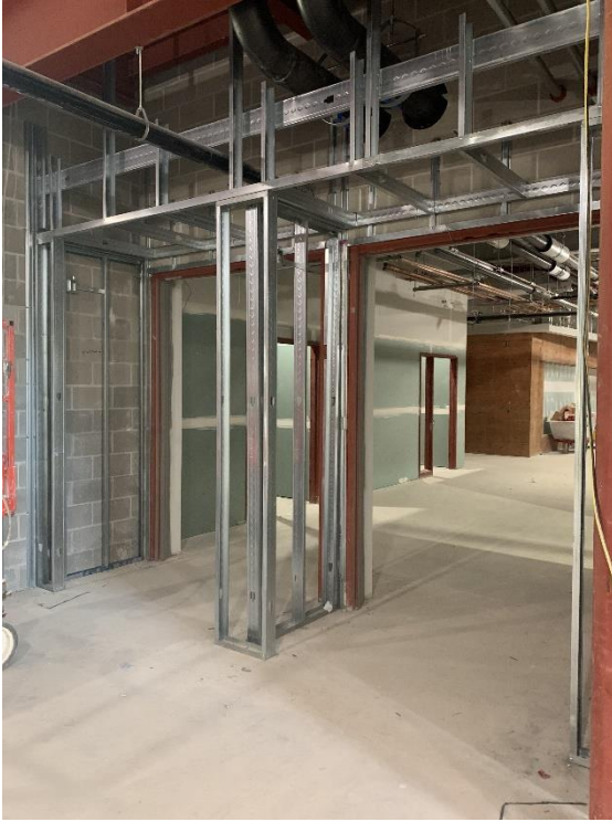
38. Area 3 – Metal stud framing and plywood backup install in first floor flex café in progress.
