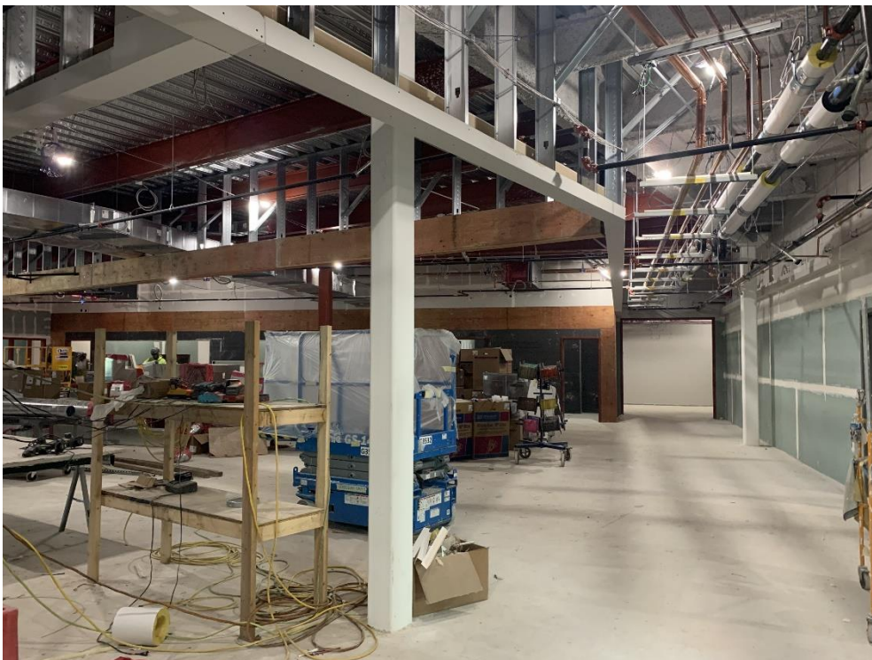
36. Area 5 – Gyp board, taping, mudding, and above ceiling MEP install first floor flex café in progress.
